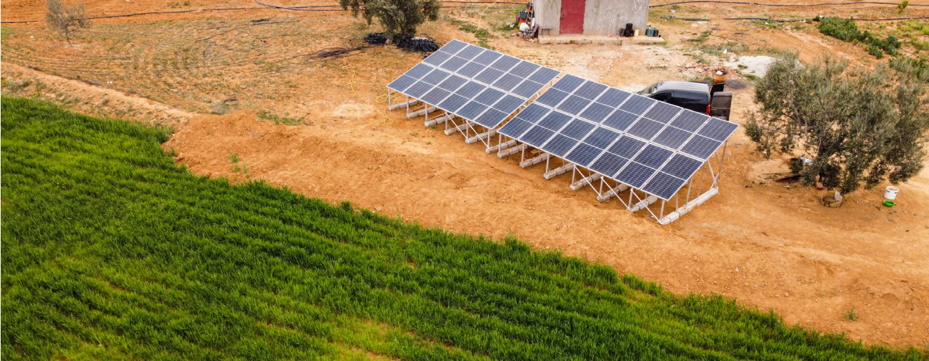
Figure 4. 10.4-kWp solar PV water pumping system for farm of Abdallah Ben Mansour in Chorbane Village in Tunisia
