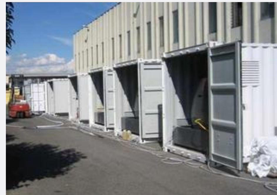
Containerised plants under construction
