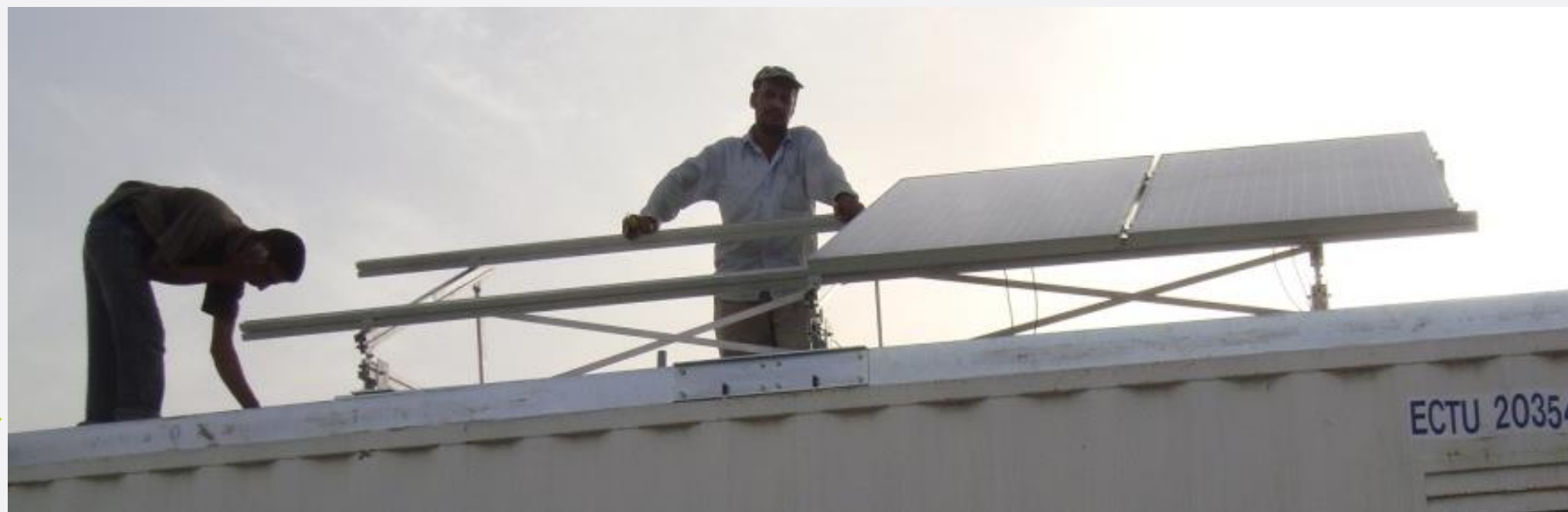
PHOTOVOLTAIC PANELS BEING MOUNTED
