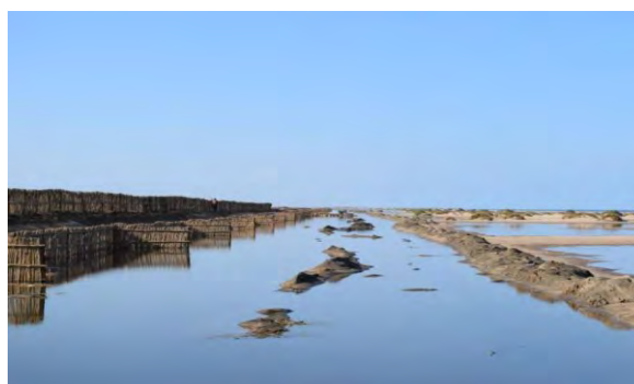
Figure 10. Constructed reed dikes for shore protection in the Delta area
